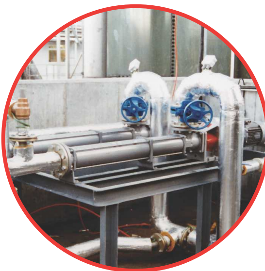
Pumping of slurry mix
